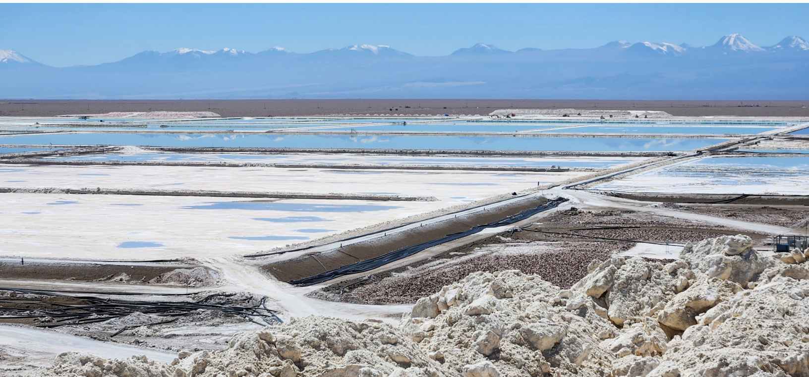
Evaporation ponds for lithium extraction in the Salar de Atacama. Photo: Terram Foundation | Cristóbal Moreno S.
